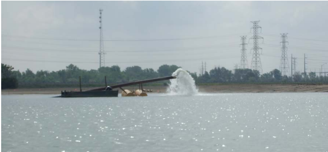
Hydraulic dredging of lake bottom sand to create islands
