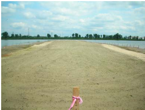
2007, immediately after construction
