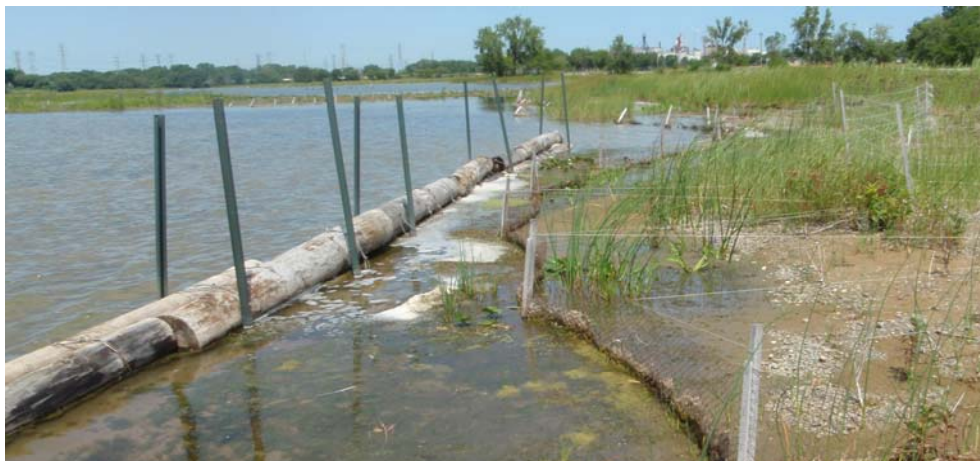
Log barrier protection of an island suffering severe erosive losses
